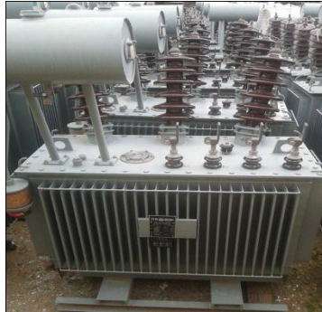
Figure2. 6 Distribution transformer
