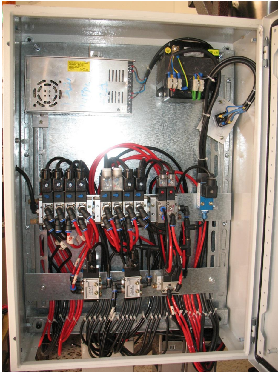
Figure (4.21): Valves Connection of the Machine
