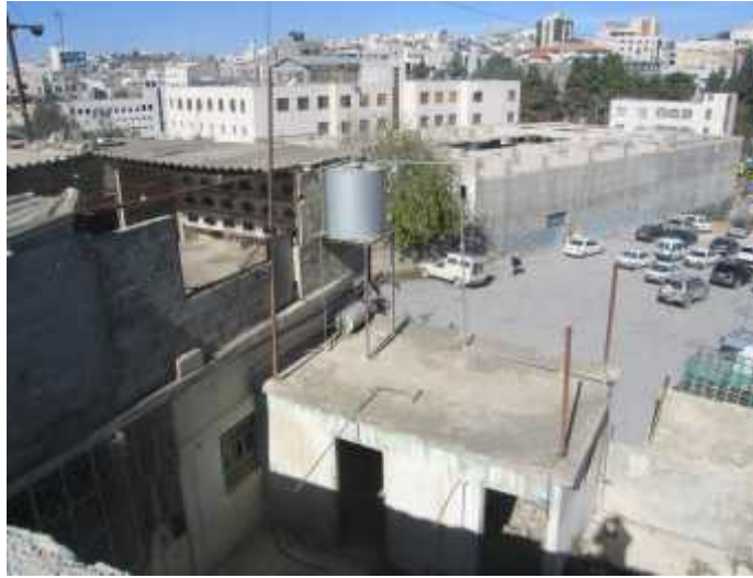
Figure 5.27 (Neglected. buildings behind the linear commercial shops, ( Source researchers, 2007)
