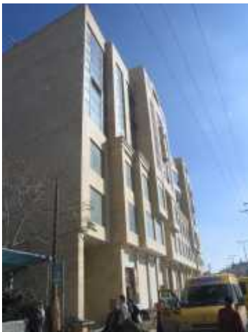
Figure 5.11 Hebron commercial center (Source researchers, 2007 )
