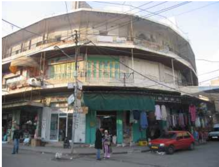
Figure 5.26 Mixed use buildings in the CBD, (Source Researchers, 2007)
