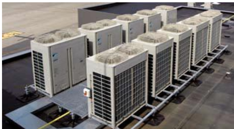
Figure (6.2) Outdoor unit
