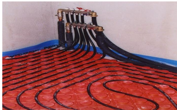
Fig (5.6) Manifolds
