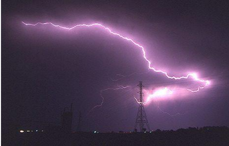
Figure 2.1: lightening strike - Transmission Tower
