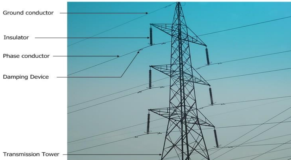
Figure 4.13: Double circuit tower
