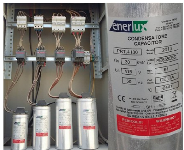
Fig 4.7 delta capacitor bank connected in transformer.
