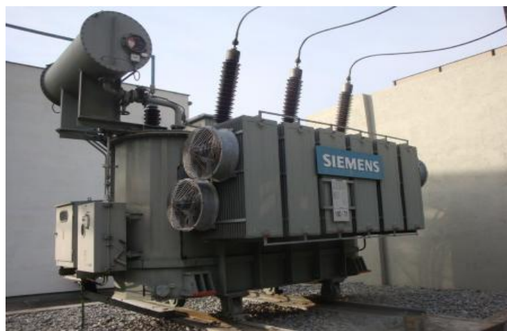
Figure 3.1: Power Transformer
