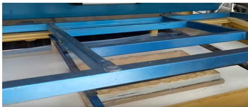
Figure 2.22: Install plastic sheet stage
