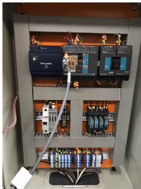
Figure 4.5: Contains of control panel
