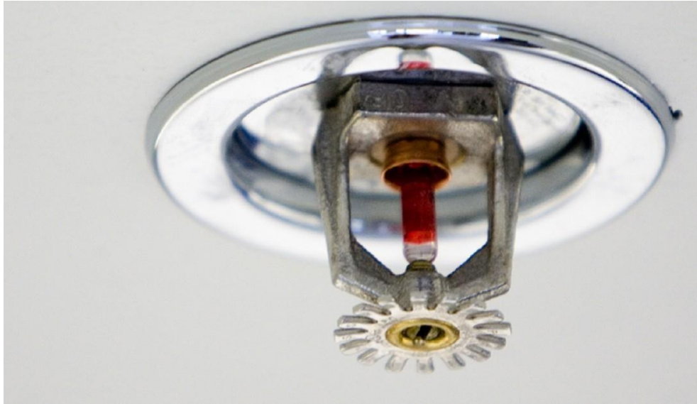
Figure 5.4: Fire sprinkler
