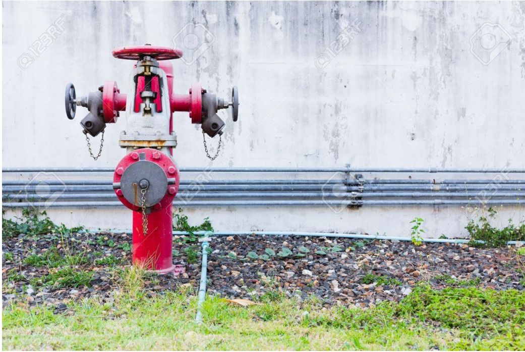
Figure 5.3: Fire hydrant system
