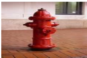
Figure (5.7) Fire hydrant
