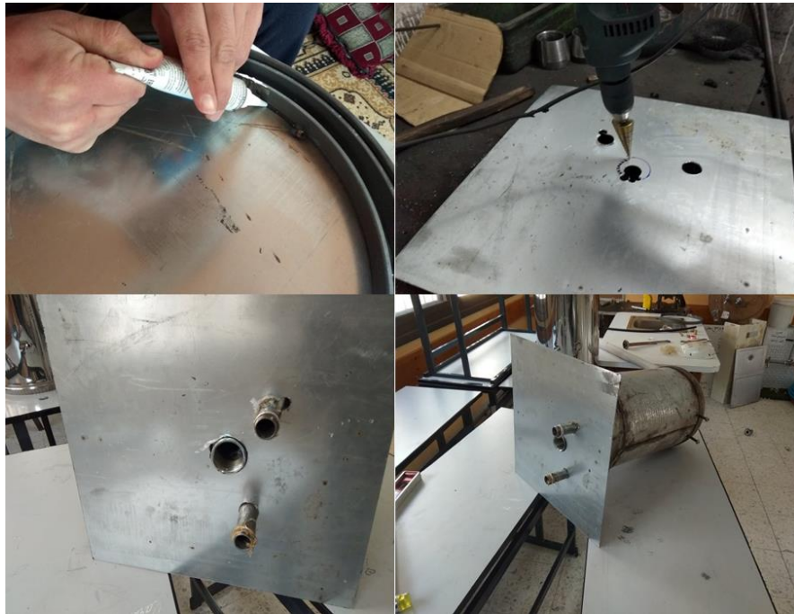
Figure (3.6) Preparation Lower Base for HWST using PW Design
