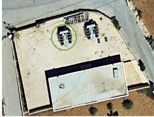
Figure 3.3: Substation #7 and Power Transformers.
