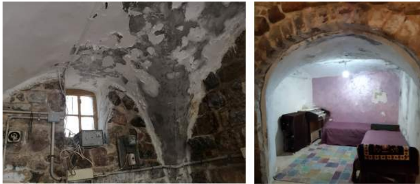
Figure 5.14: The Damp Problem (Left), The Lack of The Daylight (Right), (Researcher)
